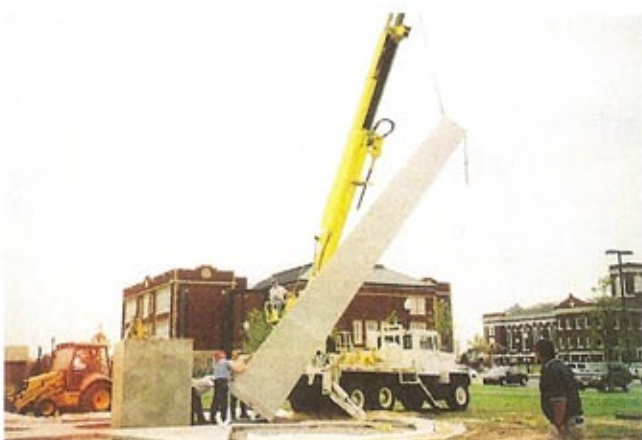
Fig. 6 — Placing the obelisk on site.
