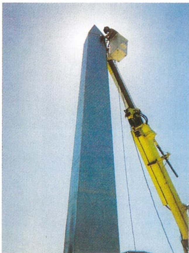
Fig. 7 — Welding on the final piece, the pyramid cap.
