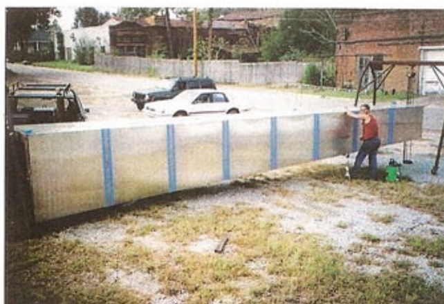
Fig. 4 — Applying the pickling gel to the weld joints.
