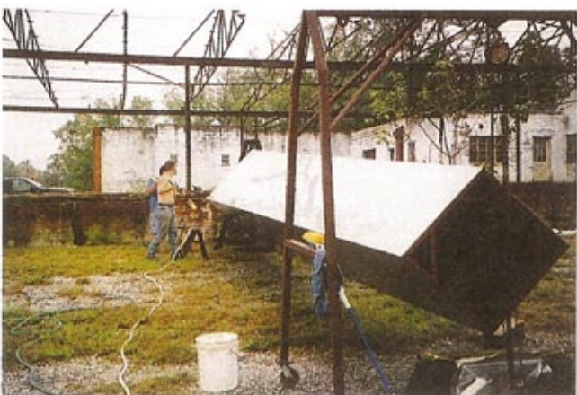
Fig. 5 — Final washing of the obelisk following application of the pickling solution. Merrill called this “the spin cycle.”
